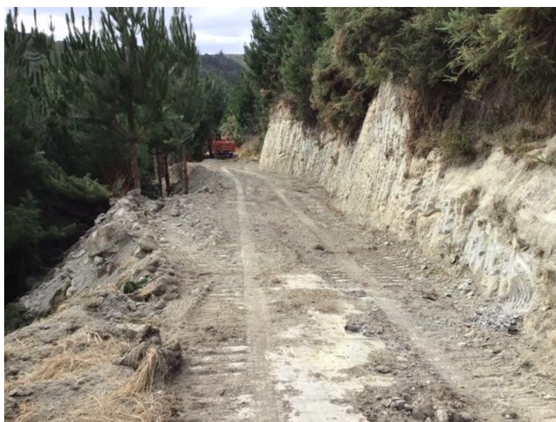
Photo 1: Track maintenance with excavator on Thompsons JV forest. Photo Josh Penn.
